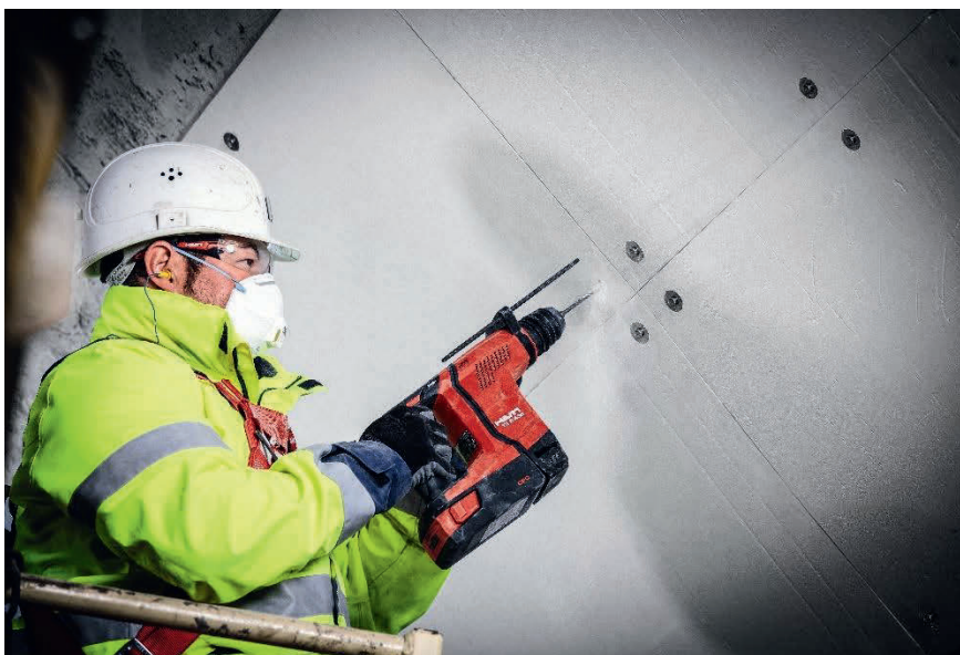
Fastening of pre-fabricated fire protection boards
